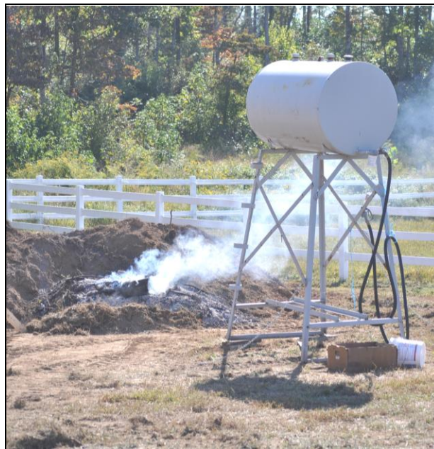
This unattended fire is within a dangerous distance to this fuel storage tank.
